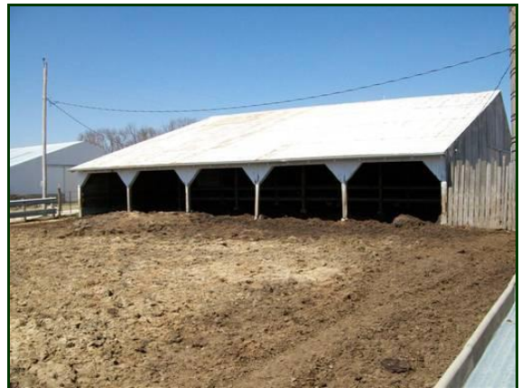
Open Front Cattle Shed
